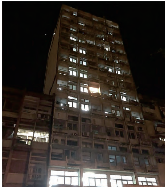
Fig. 2: The towering dormitory. At night, it has the overwhelming feeling of a haunted mansion.
